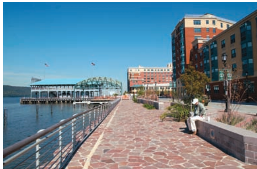
A former brownfield site on the Hudson River in Yonkers now offers housing, a promenade and recreation.
